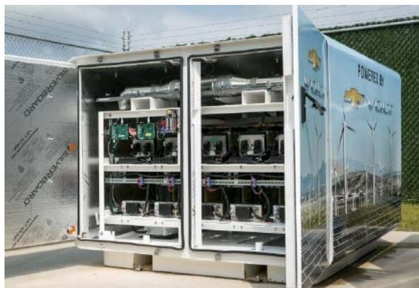
Figure 6 Energy Storage Facility Using Chevrolet Volt Batteries
